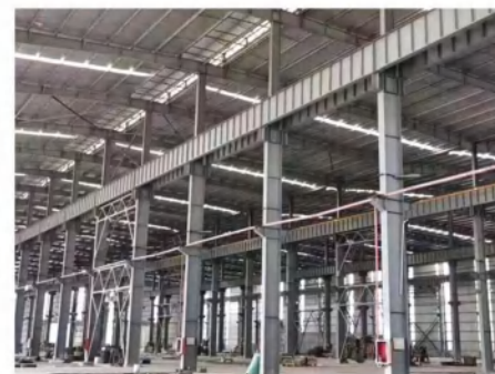
钢结构厂房 STEEL STRUCTURE WORKSHOP
