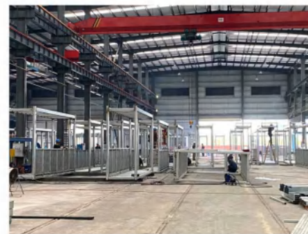
钢结构加工 STEEL STRUCTURE PROCESSING
